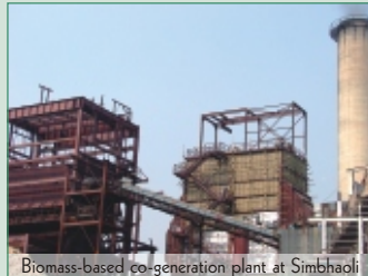
Biomass-based co-generation plant at Simbhaoli
