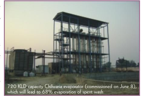
720 KLD capacity Chilwaria evaporator (commissioned on June 8), which will lead to 68% evaporation of spent wash
